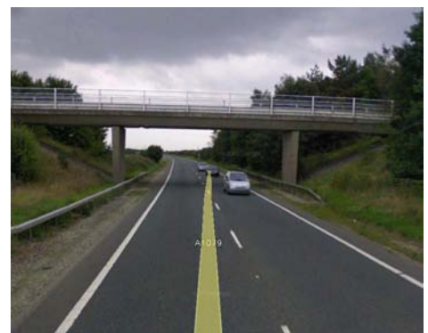
ABOVE: Road View Of Poplar Farm Bridge (5.28m)
