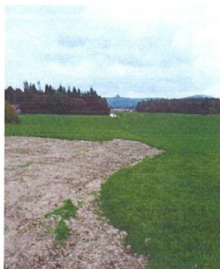
Figure 4.21 Example of cable installation swathe after topsoil reinstatement
