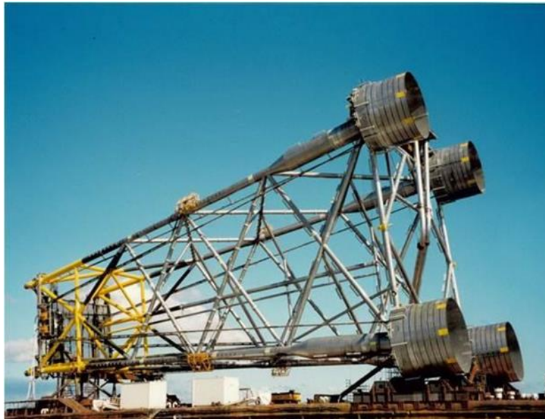
Figure 3.10 Example of a suction bucket multileg foundation
