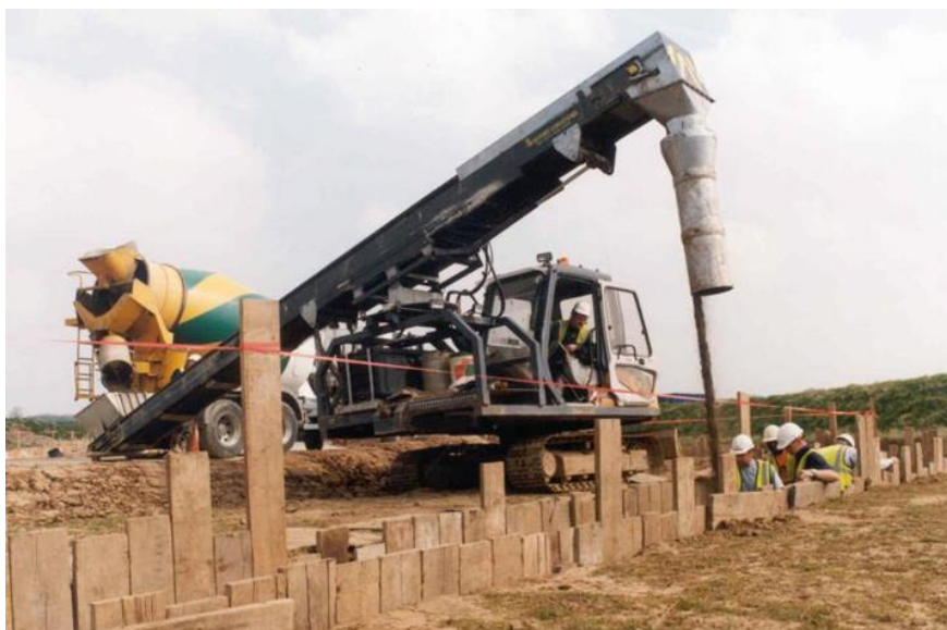
Figure 4.20 Example of a cement bound sand delivery
