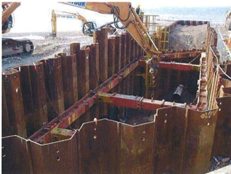
Figure 4.2 Example of a sheet piled cofferdam being installed on a beach
