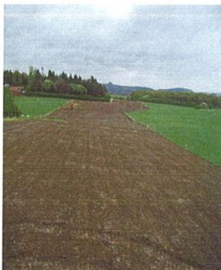
Figure 4.21 Example of cable installation swathe after topsoil reinstatement
