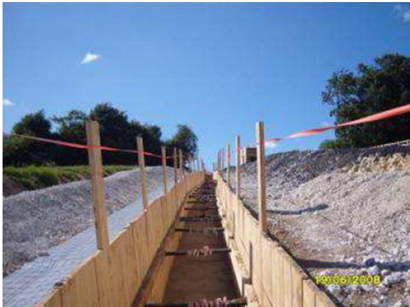
Figure 4.8 Example of close timbered trench
