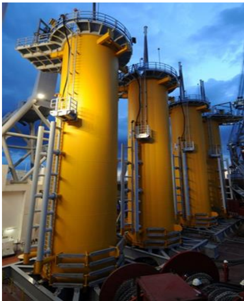
Transition pieces ready for installation (left) and transition piece being installed (right). By CHPV, courtesy of Scira Offshore Energy
