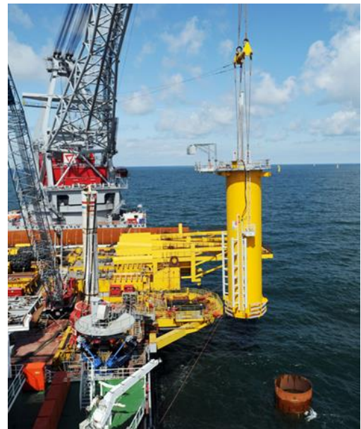
Transition pieces ready for installation (left) and transition piece being installed (right). By CHPV, courtesy of Scira Offshore Energy
