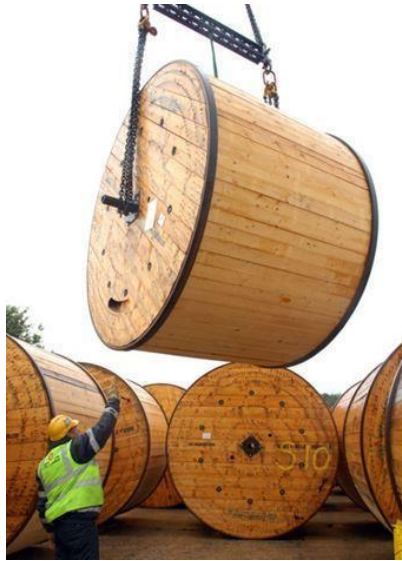
Figure 4.19 Example of a cable drum delivery to cable storage area
