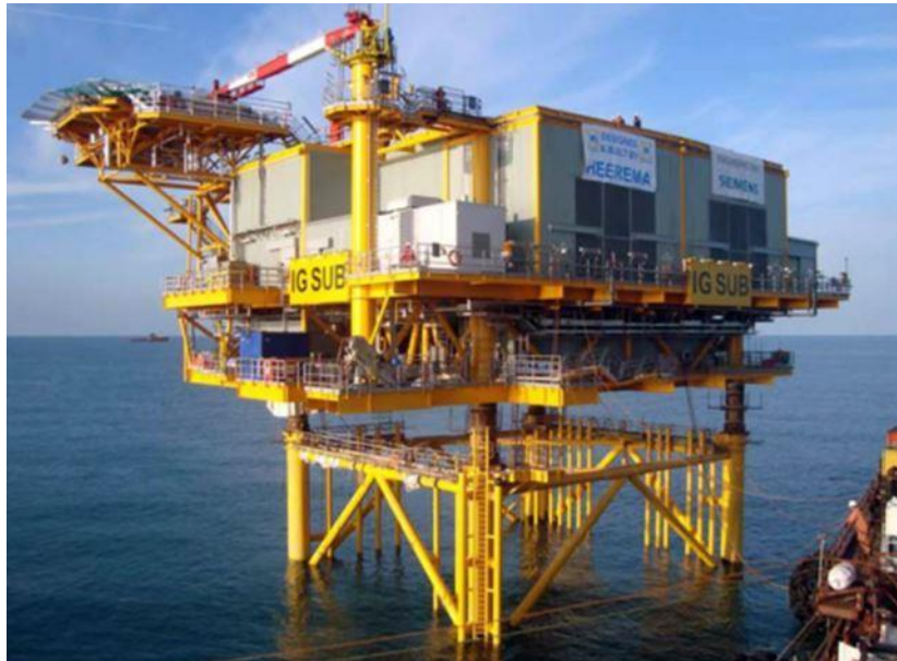
Figure 3.26 Typical offshore collector platform design
