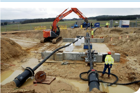
Example of landfall works
