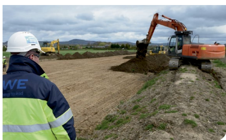
Onshore cable route reinstatement at Gwynt y Môr Offshore Wind Farm
