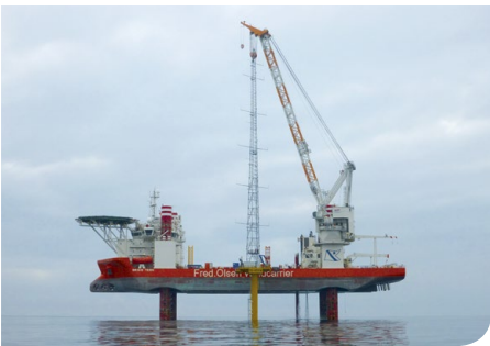
Installation of meteorological mast
