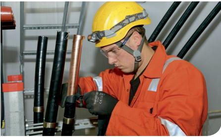
Above top: Cable laying by Team Oman Above: Tying off cables inside a turbine
