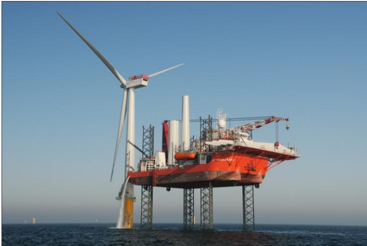
Figure 5 Turbine assembly
