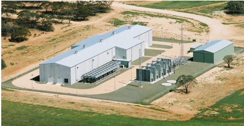
Figure 8 A typical DC-AC Converter Station at Murraylink, Victoria, South Australia (220MW)
