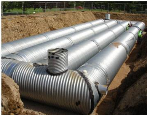
Figure 9 - Circular underground pipe tank system
