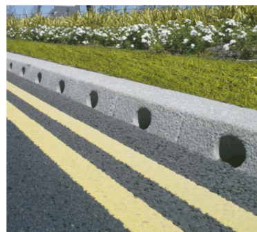
Figure 1 - Combined kerb drainage
