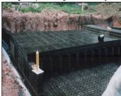
Figure 8 - Underground crate system
