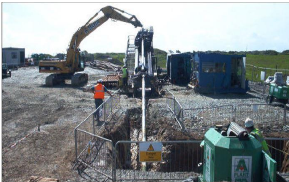
Figure 4.2 Example of typical HDD equipment
