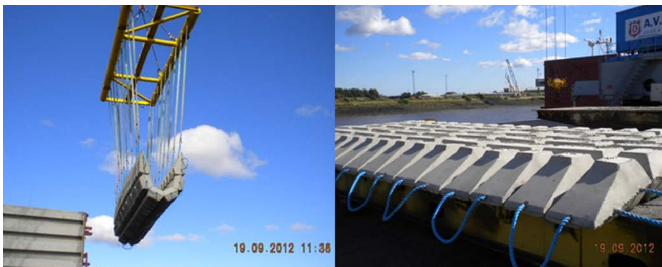
Pipeshield Bi-Flex Concrete Mattress. Courtesy of Pipeshield
