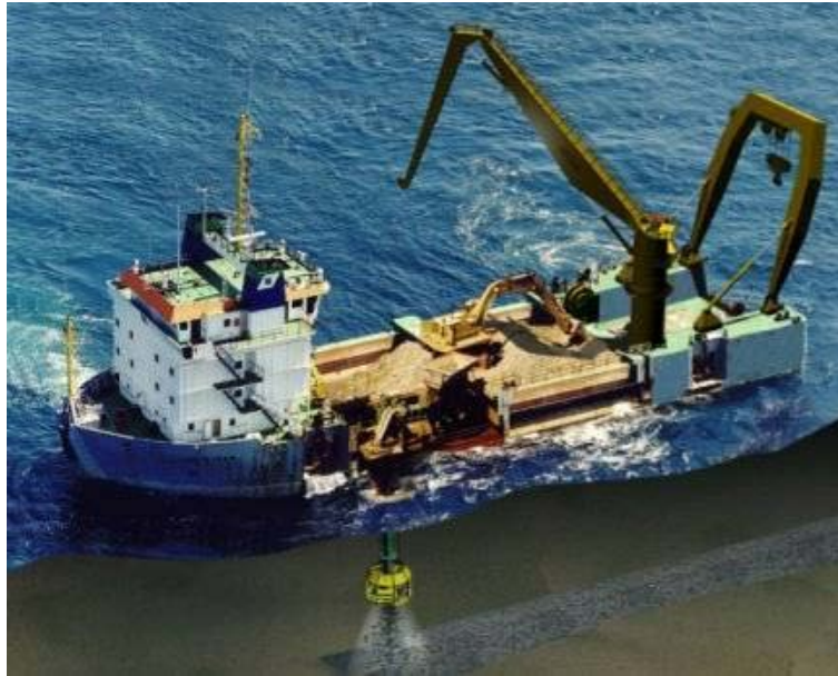
Figure 3.38 Illustrative visualisation of rock placement for cable protection
