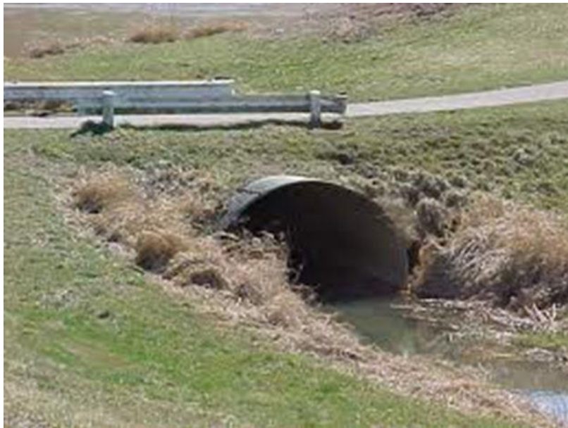
Figure 4.12 An example of a typical culvert
