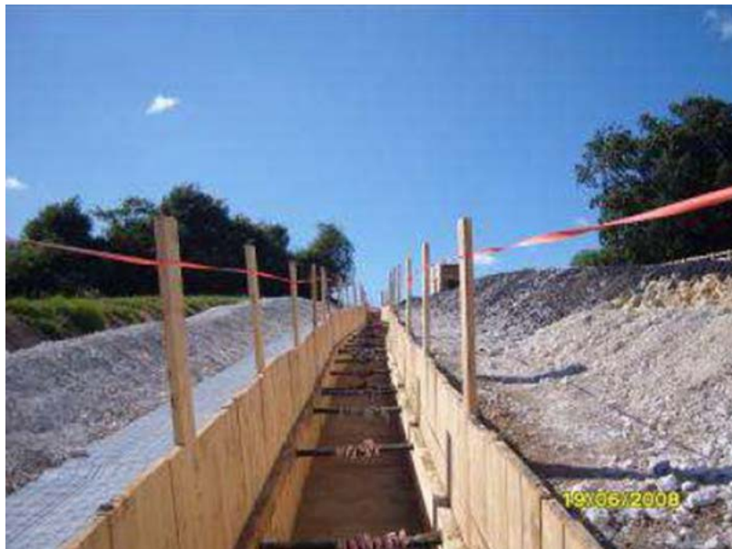
Figure 4.9 Example of close timbered trench
