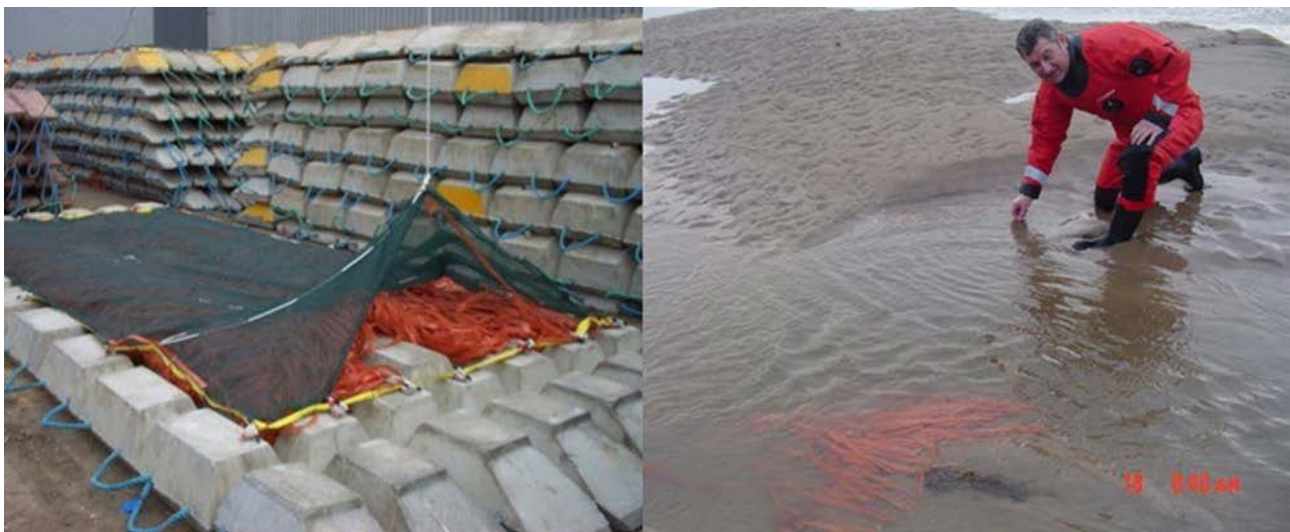
The fronds can allow self-burial in favourable conditions, by trapping sediments. Courtesy of Pipeshield
