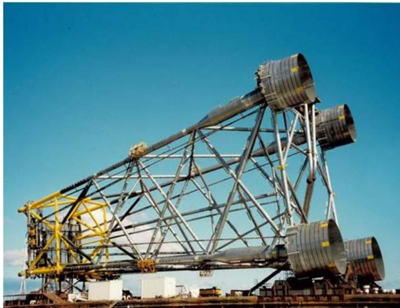
Figure 3.10 Example of a suction bucket multileg foundation
