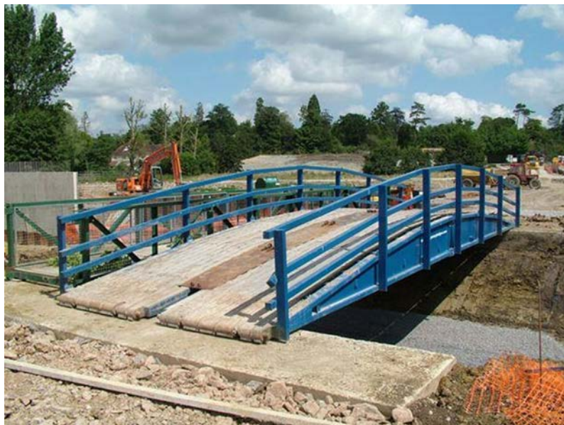
Figure 4.19 Example of a temporary vehicle bridge
