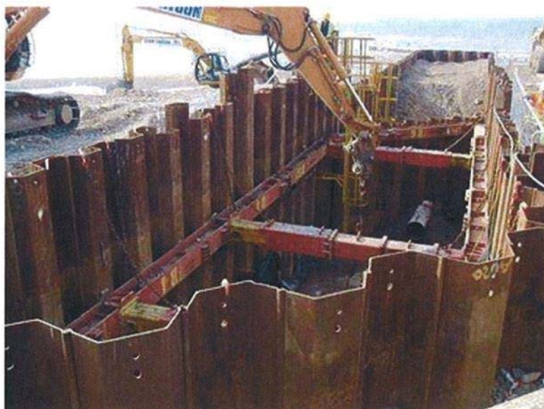
Figure 4.3 Example of a sheet pile cofferdam being installed on a beach
