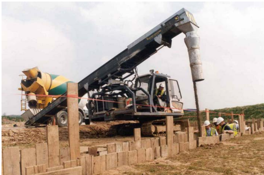
Figure 4.21 Example of a cement bound sand delivery
